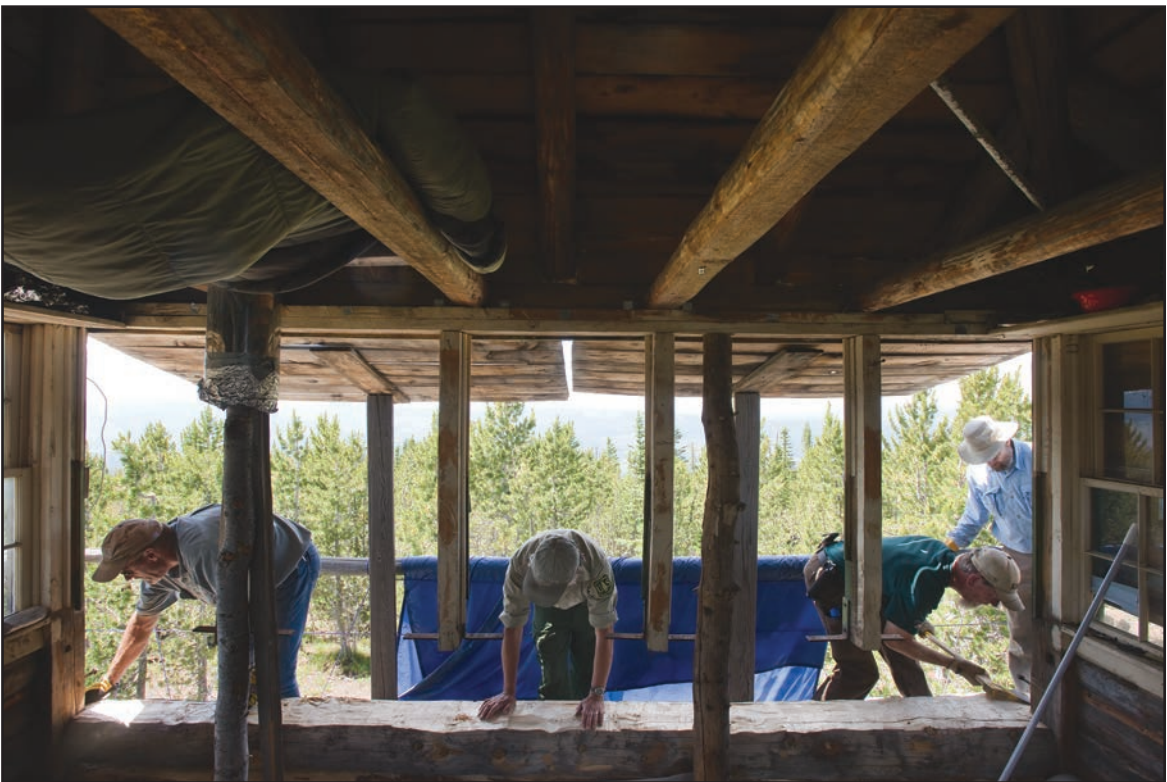
From left, Bob Beiermann, Jamie Schoen, Bill Hesketh and Jack Sterling fit a log into the western wall of the Huckleberry Fire Lookout last week in the Teton Wilderness. They worked with Bridger-Teton National Forest staff for five days to replace the wall.
