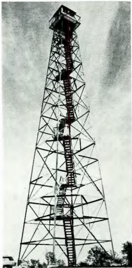
This completed tower is located near Winchester.
