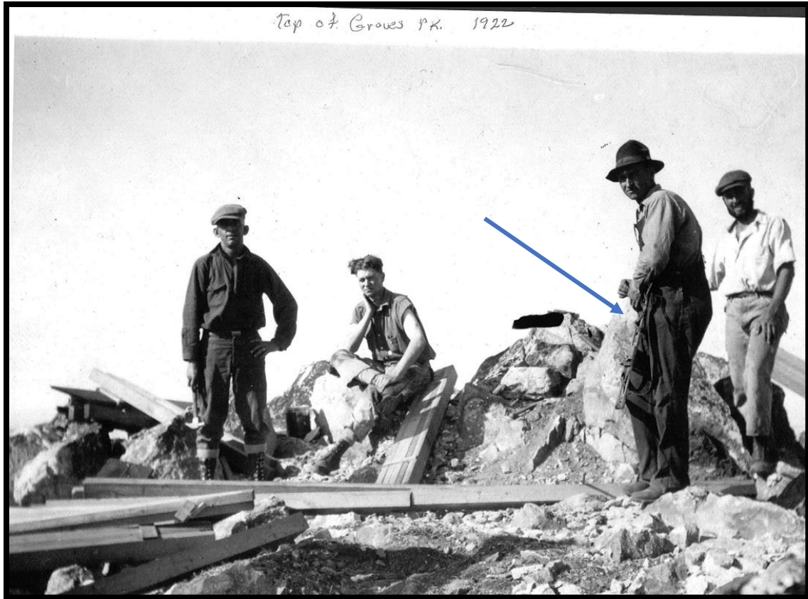
Grave Peak in 1922. Notice the lumber and back board in one of the man's hands. It appears that the men were packing lumber to the peak for construction of the lookout. Bill Bell photograph, USFS collection.
