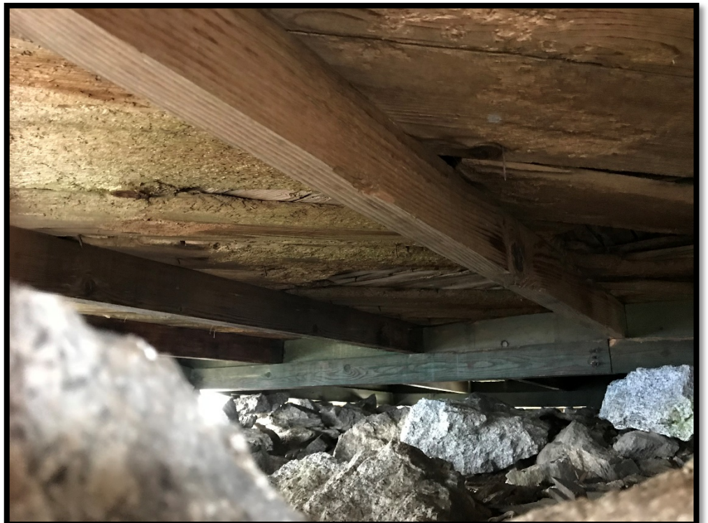
Photo 18-227 View of floor joists and subfloor. Photograph taken from under building. Direction: NA
