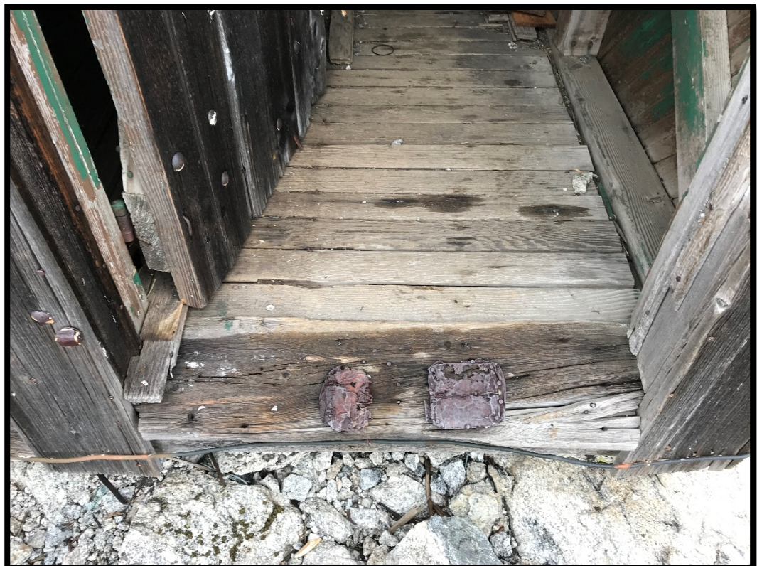
Photo 18-223 Close-up of door threshold. Direction: NA
