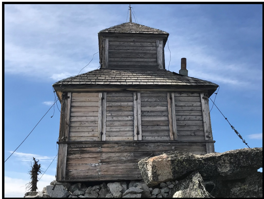
Photo 18-213 North elevation. Direction: south
