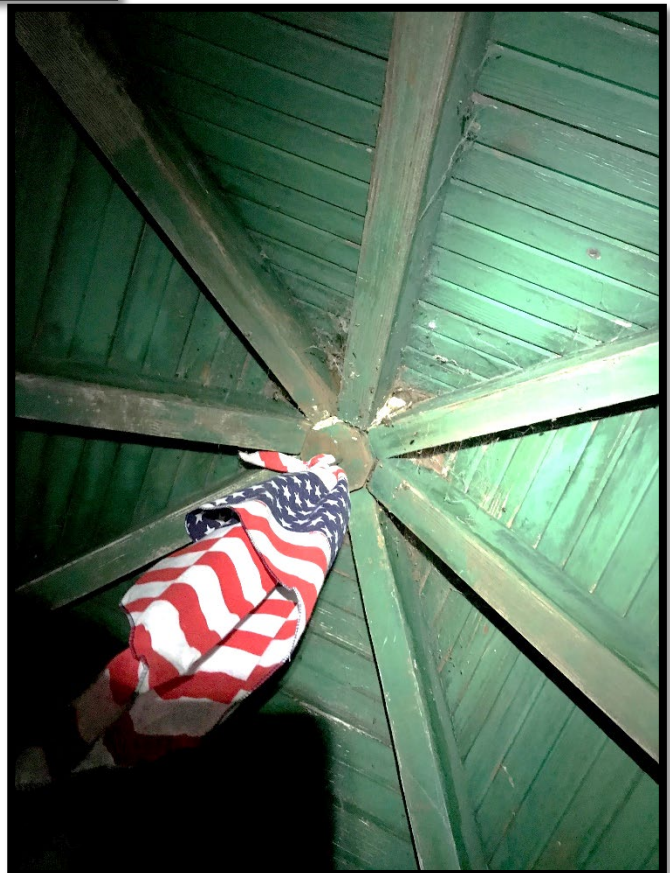
Photo 18-219 Looking up at the roof of the cupola from within the lookout. Direction : NA
