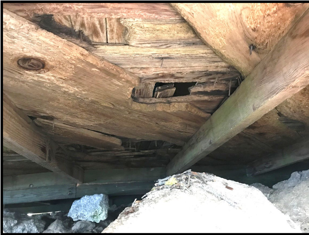
Photo 18-226 View of floor joists and deteriorated subfloor. Photograph taken from under building. Direction: NA
