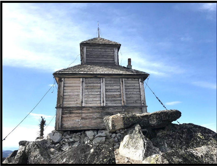
Photo 18-212 Grave Peak Lookout. North elevation. Direction: south
