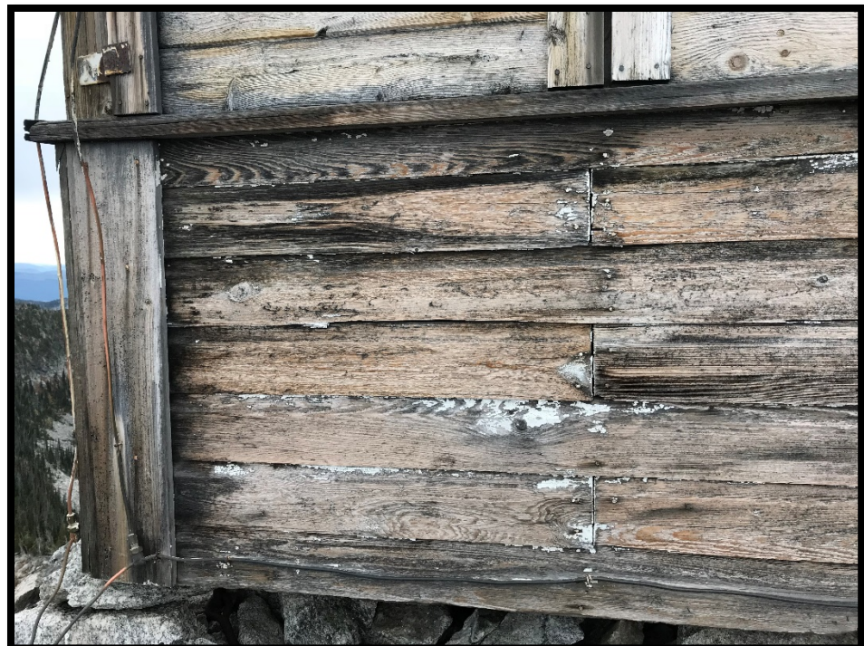
Photo 18-221 Close-up view of shiplap siding. Direction : NA
