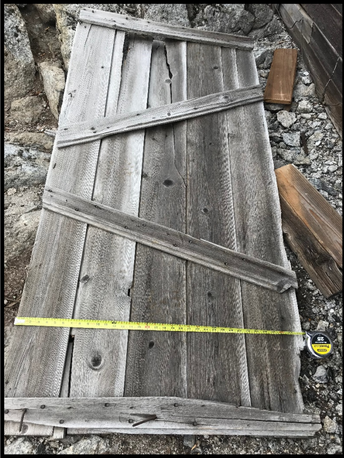
Photo 18-224 This appears to be an original window shutter that was left laying on the ground. Direction: NA
