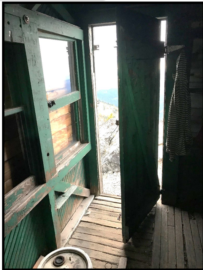
Photo 18-217 Looking at door and opening on the south elevation. Photo taken from inside the lookout. Direction: south
