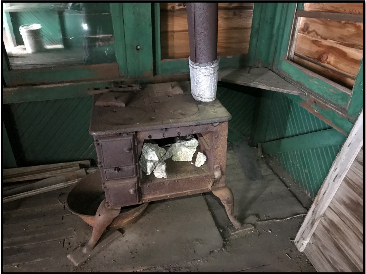
Photo 18-228 Interior view of lookout and wood stove. Direction: NA
