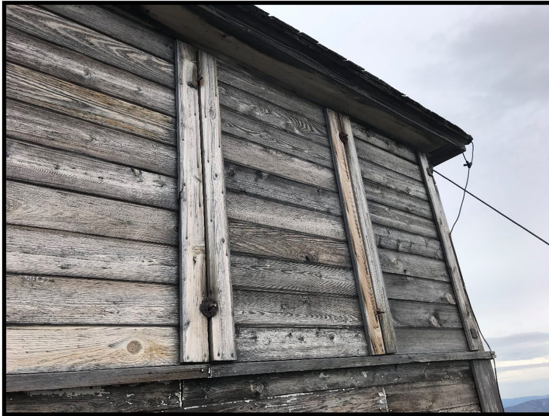
Photo 18-222 Close-up of window shutters built in 1998. Direction: NA
