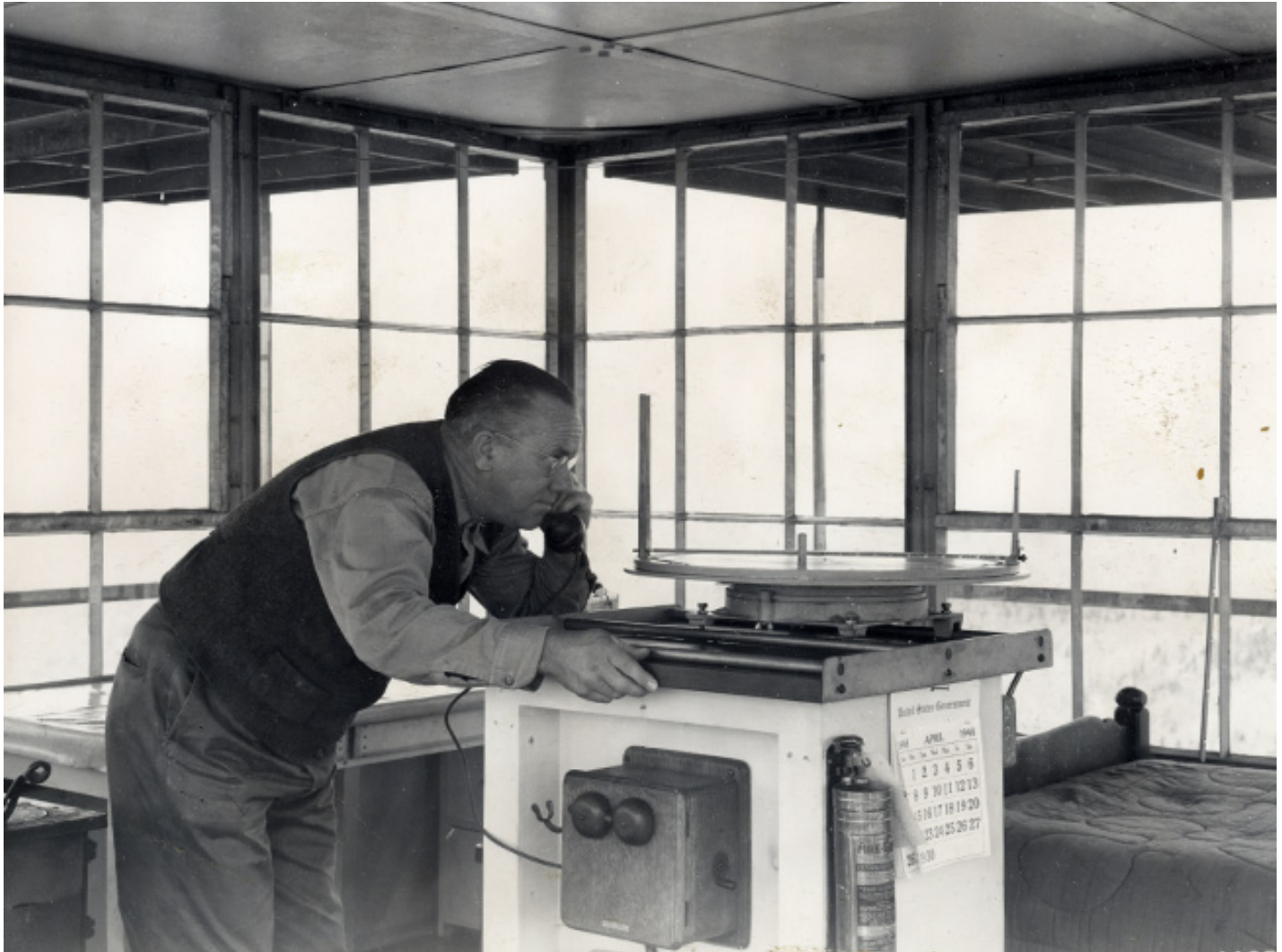
Interior of Mikes Knob Tower showing lookout Charles Dobson using his Osborne Fire Finder to spot a smoke in April 1946 (USDA Forest Service photo).
